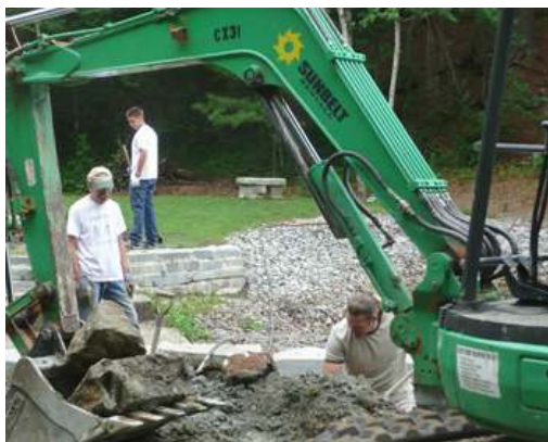
Volunteers excavate the sinkhole last summer..
